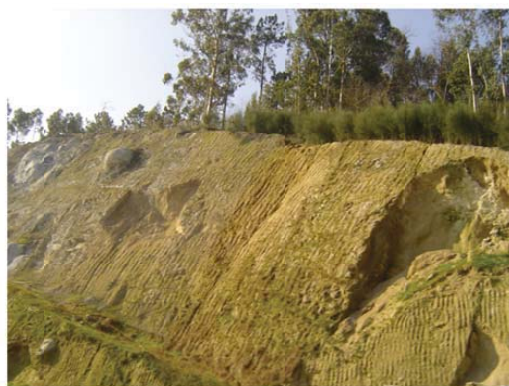
Figure 12. Variable nature with all possible weathering degrees in a granite cut on a road.
