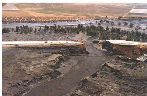
Figure 8. Failure of the Aznalcóllar dam, near Seville (Spain) on 24 th April 1998, where tailings were release to the Amargo river basin. Taken from http://www.pensandoelterritorio.com . Entered on 24 th October 2013.
